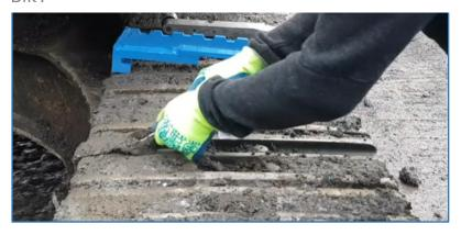
STEP 3: PUT THE BIGGER PART ONTO THE PAD AND FIX IT WITH THE SMALL PART, USING THE SCREWS
